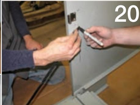
Using the previously made markings, the strap is fully extended and the mounting hole is marked with a Sharpie.
